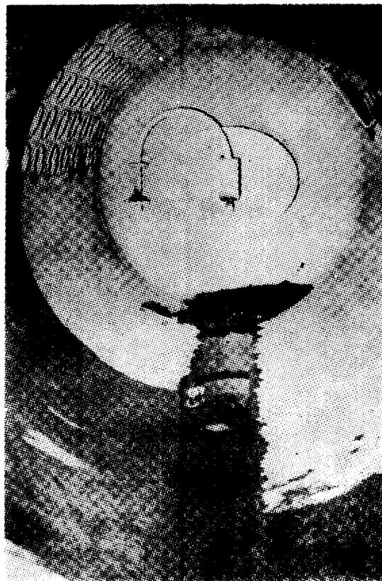
Fig. 2. When plant switched from phosphate to chelant clean-up program, the improvement was quite dramatic. Note scale in rear removed after chelant cleaning (light area).
