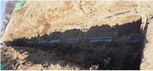
Fig. 13. Excavation result for false negative verification
