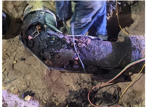
Fig. 16. Excavation result at 'Defect'
