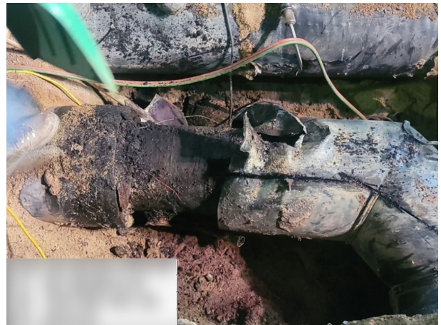
Fig. 17. Excavation result at 'Heat2'
