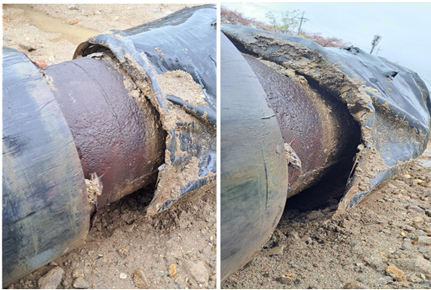
Fig. 14. Excavation result at 'DRM1'
