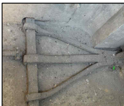
Fig. 3 Different areas of the iron bar chain with different degradation degrees.
