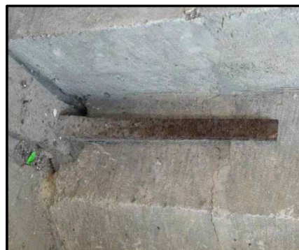
Fig. 3 Different areas of the iron bar chain with different degradation degrees.
