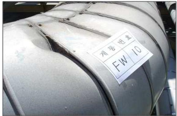
Fig. 1. Pictures of damaged fixed-insulation.
