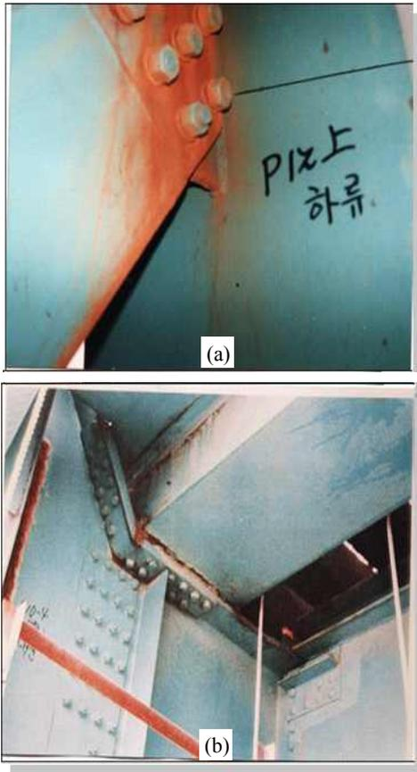
Fig. 6. Galvanic corrosion because of dew water at bolt connection inside of painted box girder.
