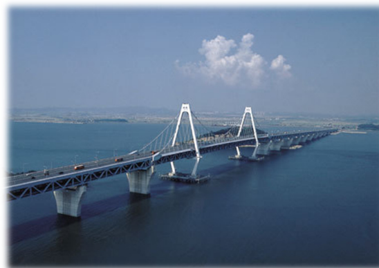
Fig. 1. The Yeongjong Grand Bridge.
