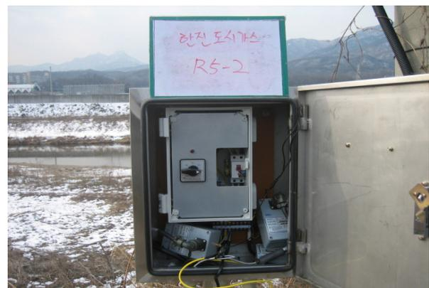
Fig. 4. A picture of distributed ICCP in the field
