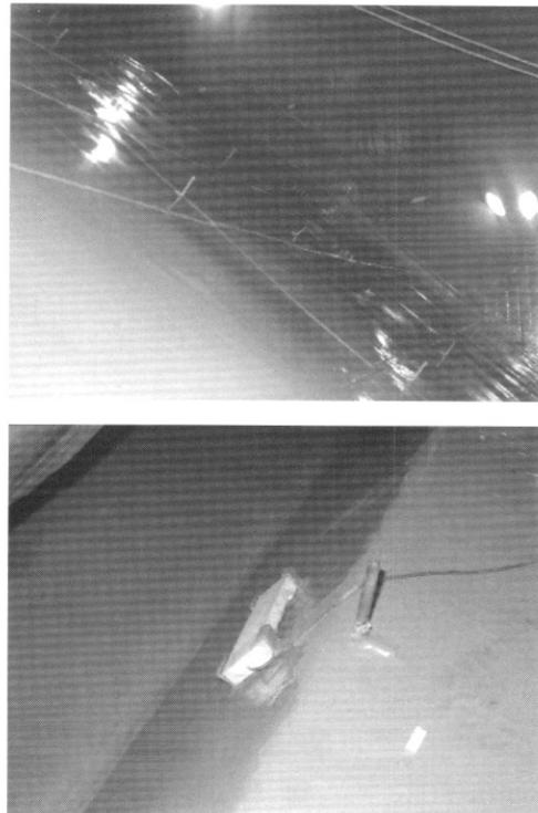
Fig. 8. Application of epoxy Novolac coating with CP anodes in FGD system
