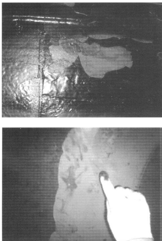
**Fig. 9.** Locally peel-offs and cracks occurred in high temperature gas
