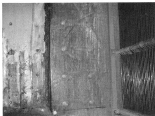
Fig. 1. Severe corrosion damages in FGD facilities
