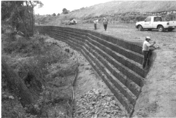
Fig. 1. Installation of geogrids
